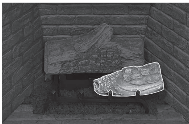
Figure 78: Log Set Installation - Step 2
