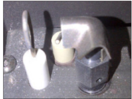
Figure 23: Correct Pilot Position
