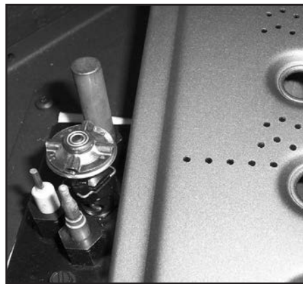
Figure 15: Ignitor assembly beside the burner.
