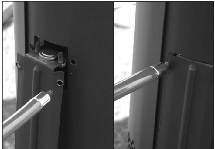
Figure 47: Spill switch installation.
